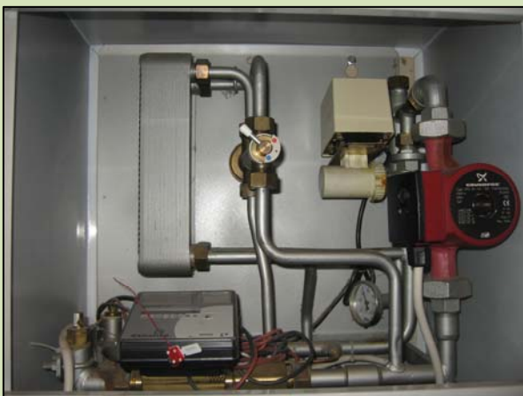
Example of an installed household heat exchanger
