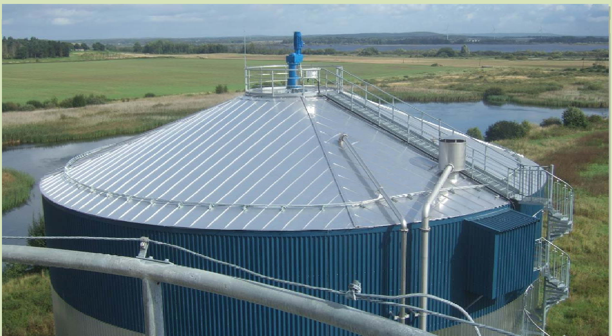
Biogas production facility located near Kristianstad, Skåne.
